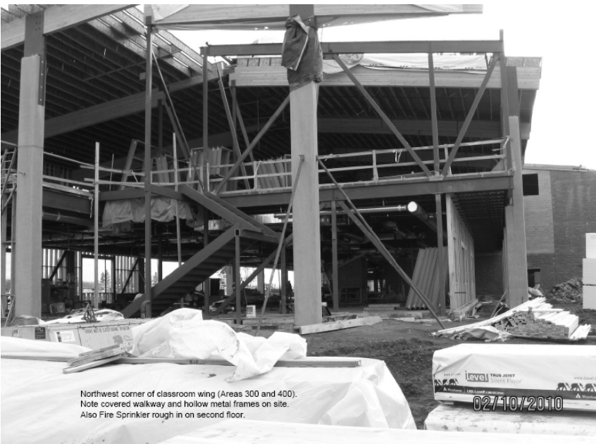
Northwest corner of classroom wing. Note covered walkway and hollow metal frames on site.
