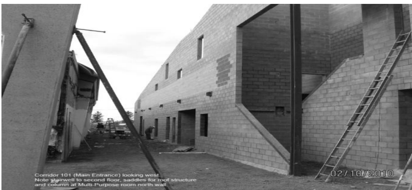
Corridor 101 (Main Entrance) looking west. Note stairwell to second floor, saddles for roof structure and column at Multi-Purpose room north wall.
