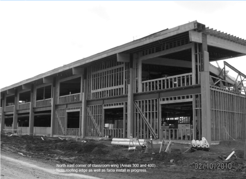
Northeast corner of classroom wing. Roof sheathing and dry-in in progress.
