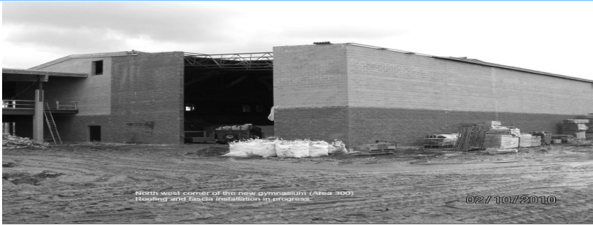
Northwest corner of the new gymnasium. Roofing and fascia installation in progress.
