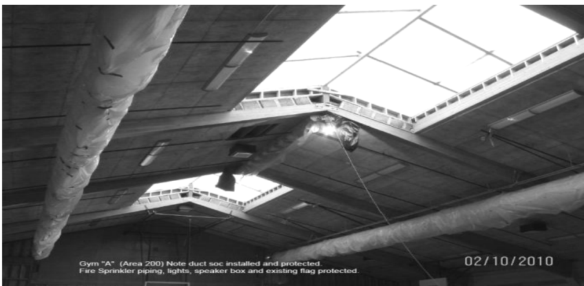
Gym "A" Note duct soc installed and protected. Fire Sprinkler piping, lights, speaker box and existing flag protected.
