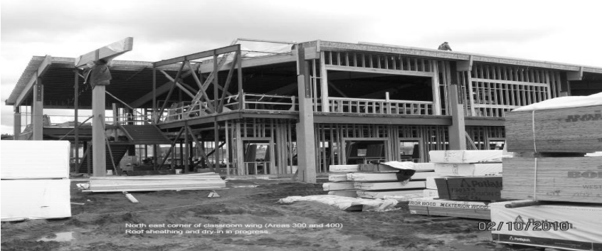
Northeast corner of the classroom wing. Roof sheathing and dry-in in progress.
